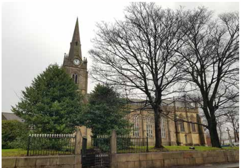
Local built character
